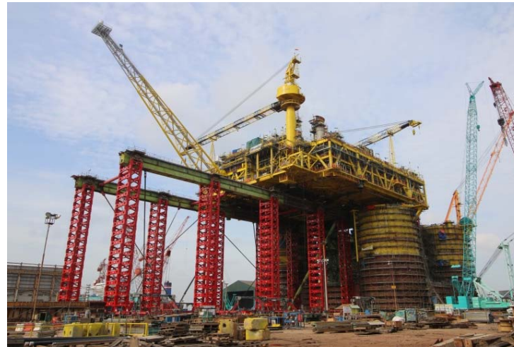
Figure 9-10: The Mega Jack is a modular system with 5,200 tonnes jacking capacity per tower. When installing more towers loads up to 100,000 tonnes or more are achievable.
