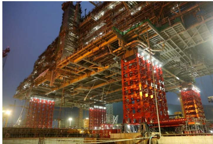
Figure 4: Mega Jack is a special jacking system capable of lifting offshore rigs with weights up to 60,000 tonnes.
