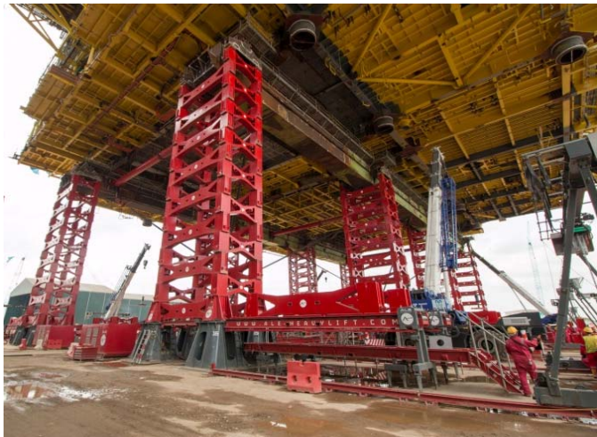
Figure 9-10: The Mega Jack is a modular system with 5,200 tonnes jacking capacity per tower. When installing more towers loads up to 100,000 tonnes or more are achievable.
