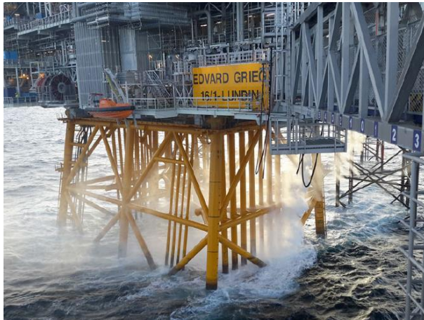
Picture 15: For the Edvard Grieg platform jacket, Dillinger delivered 12,400 tonnes of thermomechanically rolled steel of the grades S355G10+N/+M, S420G2+M and S500G2+M.
