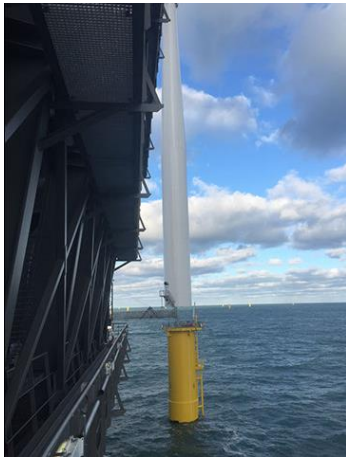
Picture 17: Wind turbines with a rotor diameter of 130 meters were installed on transition pieces made of Dillinger steel.
