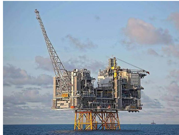
Picture 16: The 22,500 ton topside module of the Edvard Grieg platform, which is equipped with highly complex technology, 100-person living quarters and a helicopter deck, is built on a foundation structure made of Dillinger steel.
