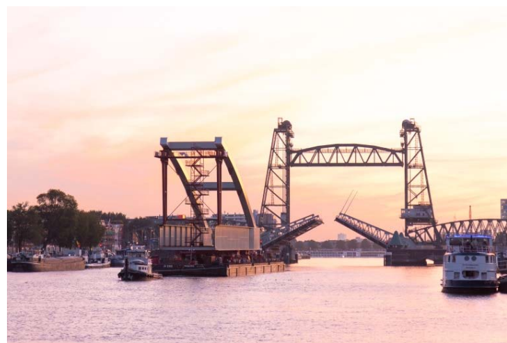
Picture 12: The combination segment of the eastern bridge deck and arch on the way to the assembly site.
