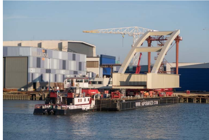
Picture 9-10: The eastern bridge deck and arch were prepared for transport on the yard premises of Hollandia.
