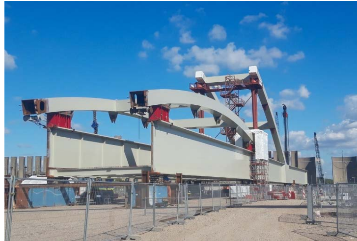
Picture 18: Assembly of the various sections took place on the assembly area close to the final site.
