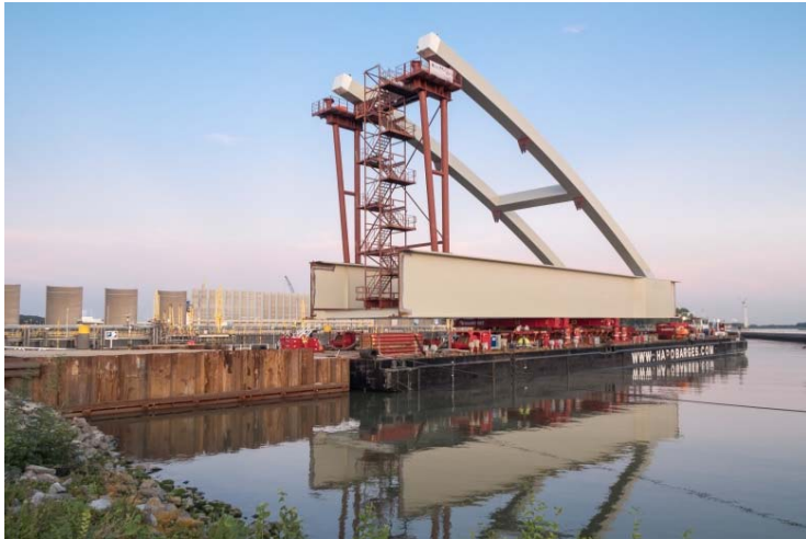
Picture 13: The combination segment of eastern bridge deck and arch section upon arrival at the assembly site.
