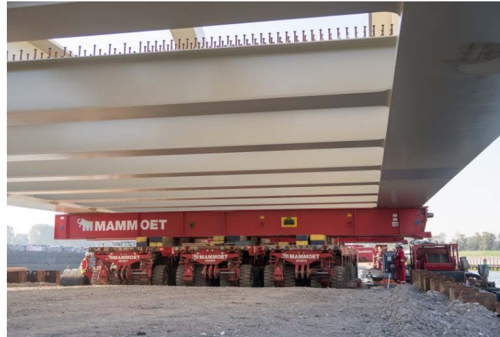
Picture 14: The assembly of the eastern bridge deck and arch section.
