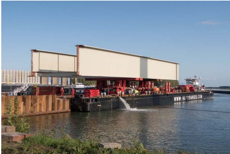
Picture 17: The completed eastern approach span is transported to the assembly site.
