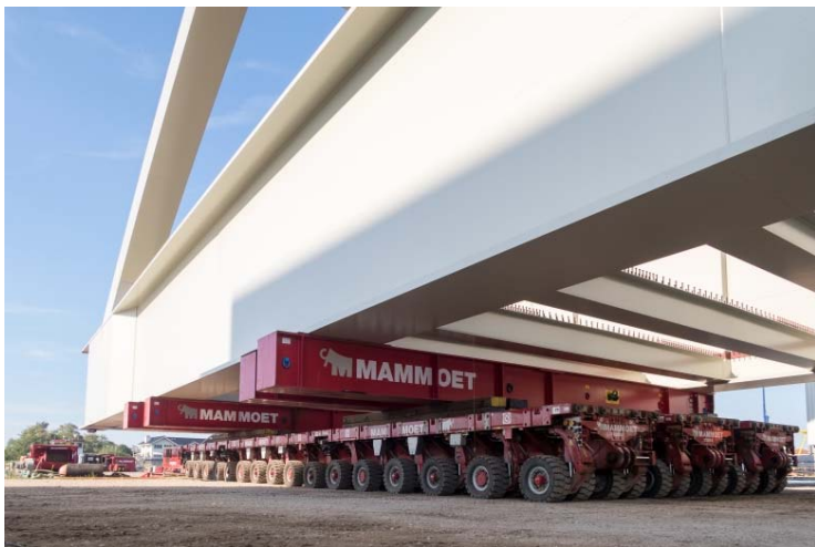
Picture 11: Loading of the combination segment of the eastern bridge deck and arch.
