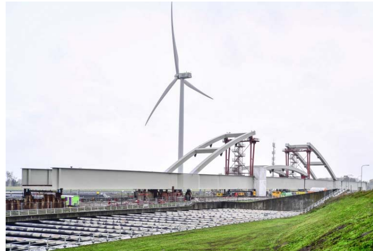
Picture 18: Assembly of the various sections took place on the assembly area close to the final site.
