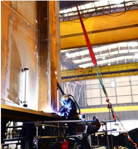
Picture 5: In the production of the elements for the main girder and all other girder plates, Hollandia benefited from the innovative weld-edge preparation of the Dillinger Heavy Fabrication Division.
