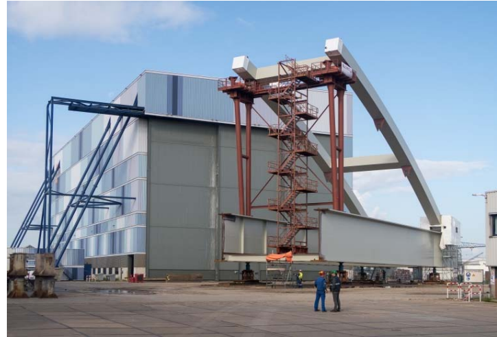
Picture 6: Four mobile cranes were used to lift the arch sections onto the respective deck sections for the components to be welded together.
