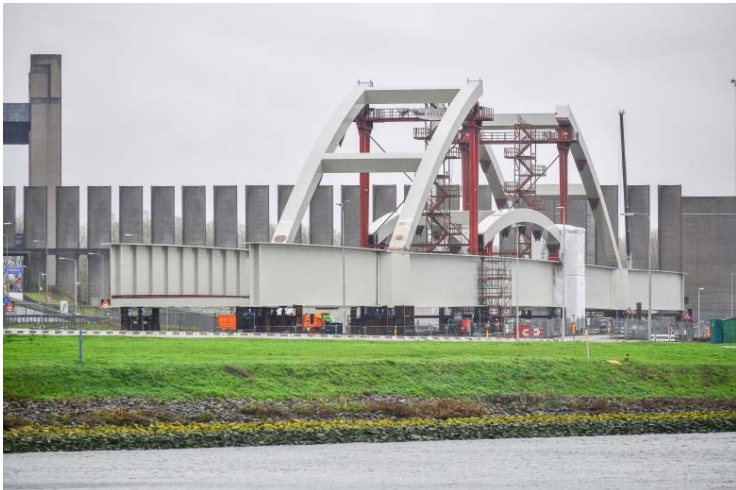
Picture 19-20: The assembly of the various sections on the assembly area close to the final site..
