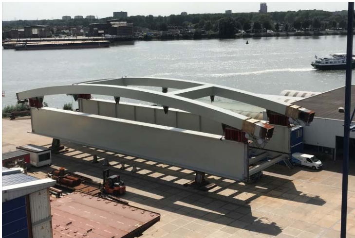
Picture 7: The combination section of the middle bridge deck and arch was prepared for the transport to the assembly area.
