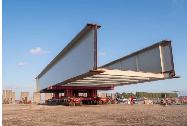
Picture 15-16: The production process was completed with the fabrication of the eastern approach span.
