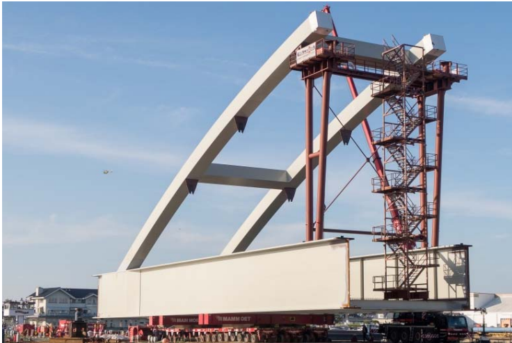
Picture 9-10: The eastern bridge deck and arch were prepared for transport on the yard premises of Hollandia.
