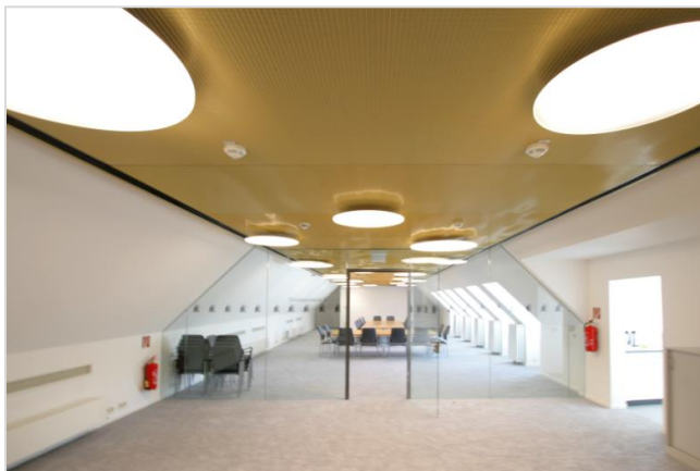
Picture 1: The ceiling system with Aluminium mesh of the type CMP-Alu 6010 ensures pleasant acoustics in the conference room.
