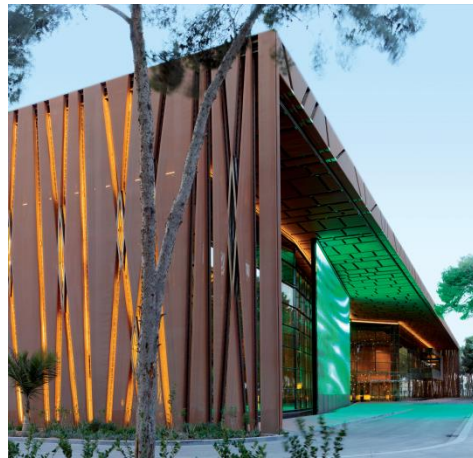
Picture 15: The shell of the Tripoli International Convention Center in Libya is made from bronze-coated stainless steel mesh type Kiwi.
