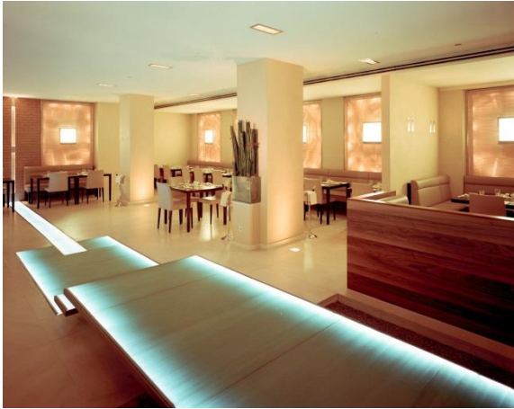
Picture 1: Multi-layer wall cladding made of backlit Mandarin bronze metallic mesh at the "Taku" gourmet meeting point in Cologne.
