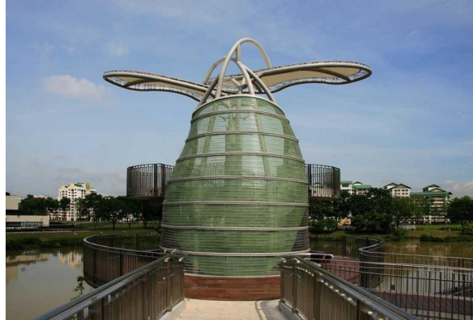
Picture 13: The semitransparent cladding made from stainless steel mesh of the Escale 7x1 type with partial green coating gives the Yishun Pond observation tower in Singapore a particular natural look.
