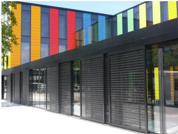
Picture 14: Escale 7x1 black-coated stainless steel spiral mesh is used to clad the cafeteria of the famous Ecole Polytechnique Fédérale (EPFL) in Lausanne, Switzerland.
