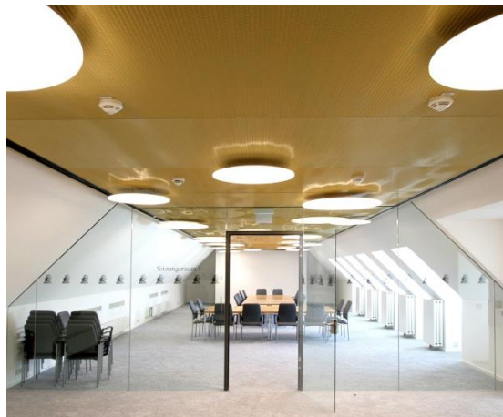
Picture 10: A golden anodised acoustic ceiling, made of the aluminium mesh type ALU 6010 gives the department "King of England" a royal feel that befits the history of the building.
