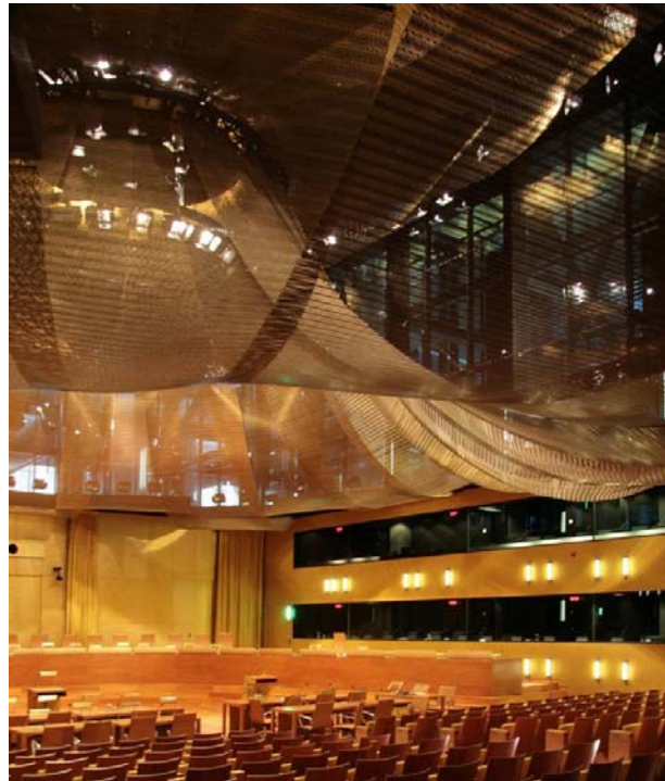
Photo 3: The elegant ceiling cladding of the Principal Courtroom is made up of 1,387 square meters of made-to-measure Escal mesh.
