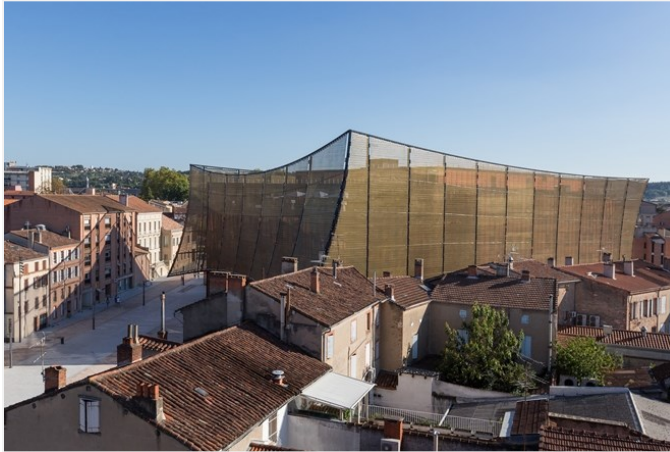
Picture 1: New attraction for Albi: The three-dimensional façade of the Grand Théâtre des Cordeliers of gold-coloured anodised aluminium mesh by GKD.
