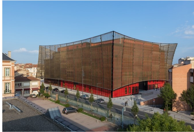
Picture 2: The spectacular construction of the woven membrane was made possible by specially developed Escalé spiral mesh by GKD.
