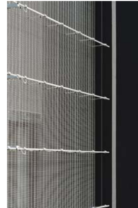
Pictures 2-4: The LED profiles are mounted at customized intervals in front of the mesh and supplied with power and image data by cables concealed behind the mesh.
