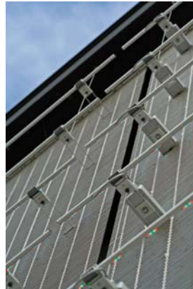
Pictures 2-4: The LED profiles are mounted at customized intervals in front of the mesh and supplied with power and image data by cables concealed behind the mesh.
