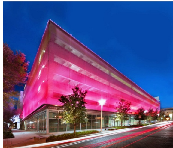
Picture 3–4: The almost 2.500 m 2 facade is clad with a total of 49 panels of stainless steel mesh of the type Helix and illuminated by coloured LED lights.
