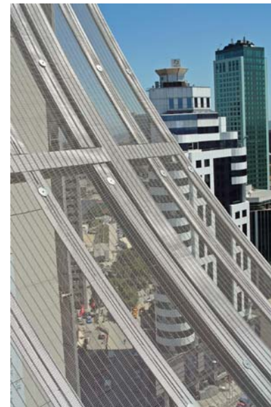
Picture 5: Elegantly undulating roof sail made of Tigris mesh at the top of the building.
