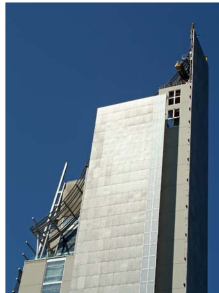
Picture 4: Shimmering Lago mesh fronts the glass façade and provides reliable sun protection.
