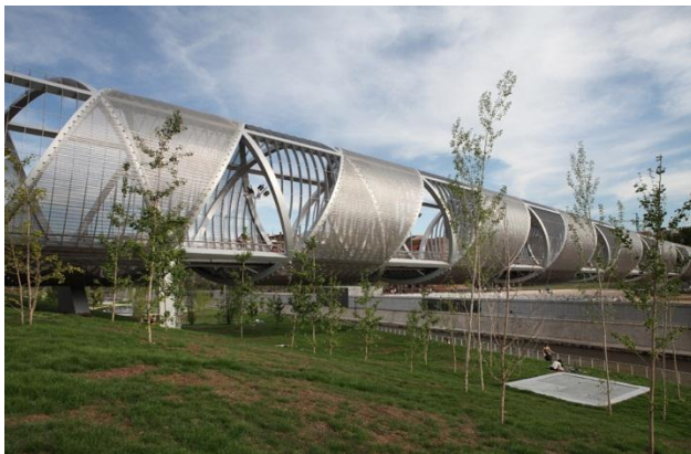
Picture 3: Stainless steel mesh type Escale surrounds the bridge in full length, creating a shimmering helix.
