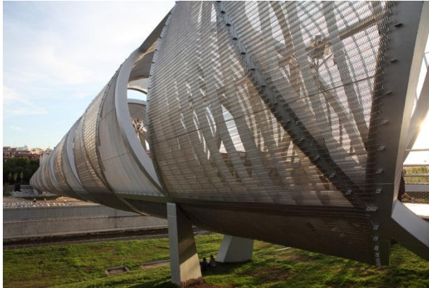
Picture 5-6: The mesh ribbon permits a natural illumination and ventilation of the bridge while at the same time offering protection from the sun.
