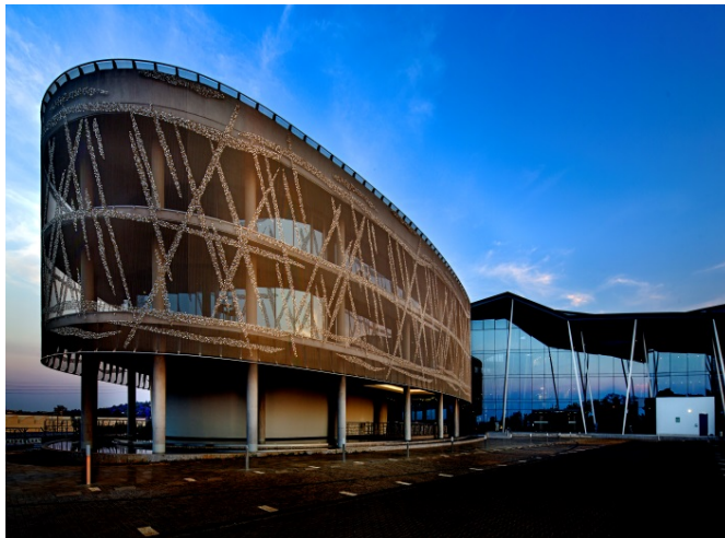
Picture 2: A total of 2,280 square meters of Omega mesh by GKD were used to create 41 panels with various widths and a height of 10.14 meters.
