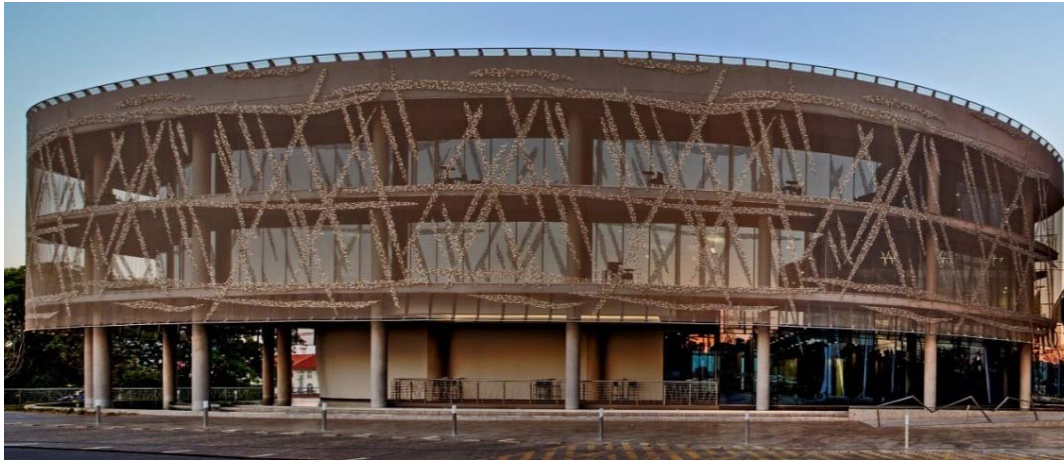
Picture 4: The ingenious interplay of more than 500,000 stainless steel buttons affixed to the woven skin by GKD creates a pattern that replicates the inscription of a Stone Age counting tool.
