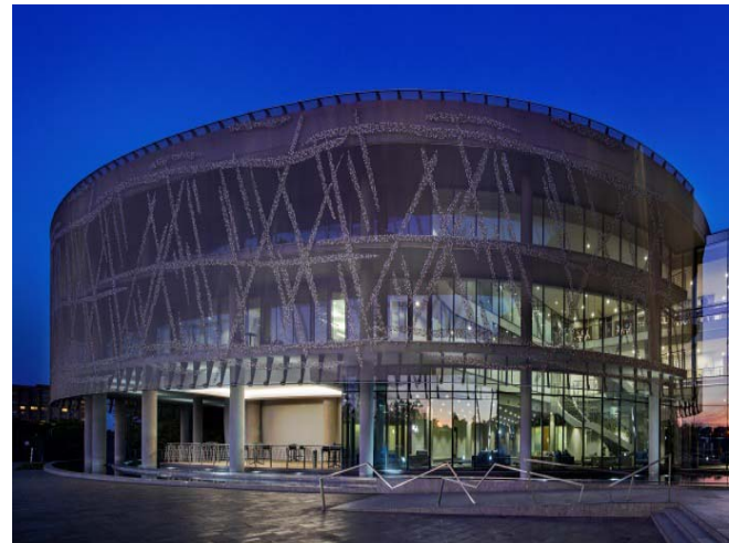
Picture 3: Thanks to its visually seamless metal mesh shell by GKD, a rotunda at the main entrance has an appearance reminiscent of a drum.
