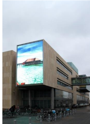
Picture 2: The MEDIAMESH®-System of type Tigris by GKD – Gebr. Kufferath AG – makes a valuable contribution to reducing solar input without compromising on light yield or visibility.
