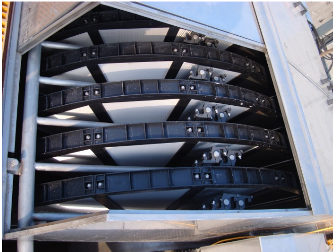
Picture 1: Installed ODW filter elements.
