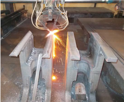
Picture 2: These notches had to be accomplished in a wide range of different cutting heights, widths and depths.
