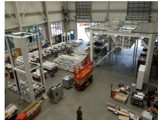
Picture 12: An extruder platform under construction
